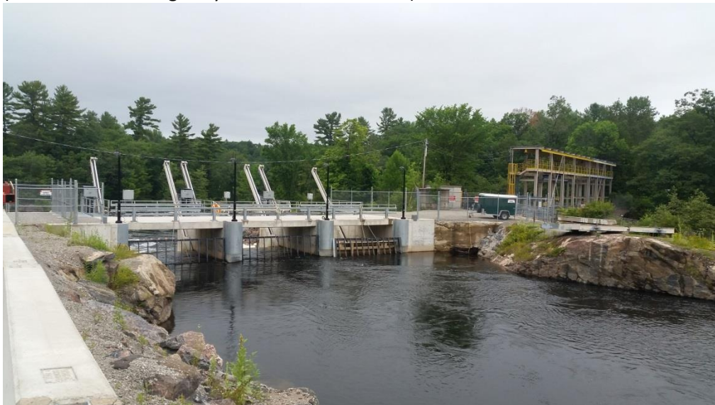
Photo 3 Wasdell Falls VLH Forebay
