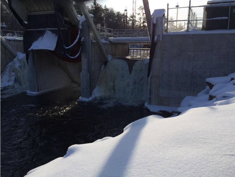
Photo 4 Ice Accumulation on downstream side of VLH Structure
