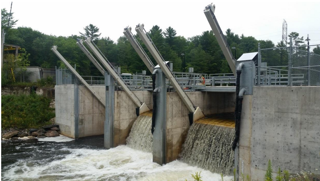
Photo 5 Wasdell Falls Downstream of VLH Structure
